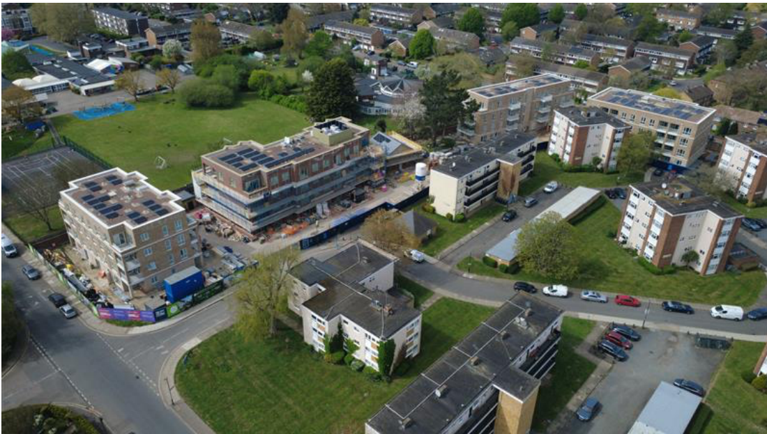
Current Progress on Site
