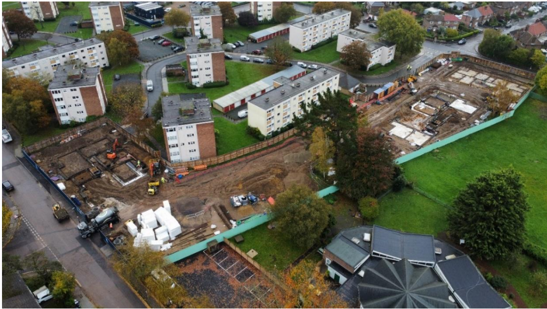
Aerial view of current site progress
