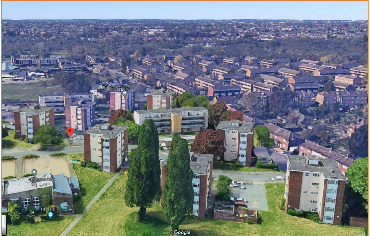
Figure 10: View of Blocks towards Woodville Road (Google 2022)
