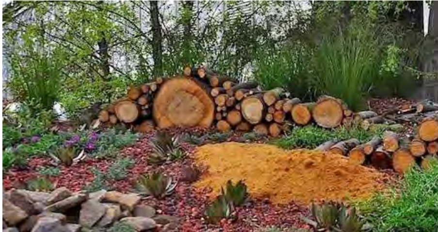
Figure 6.5 Log piles on a biodiverse roof
