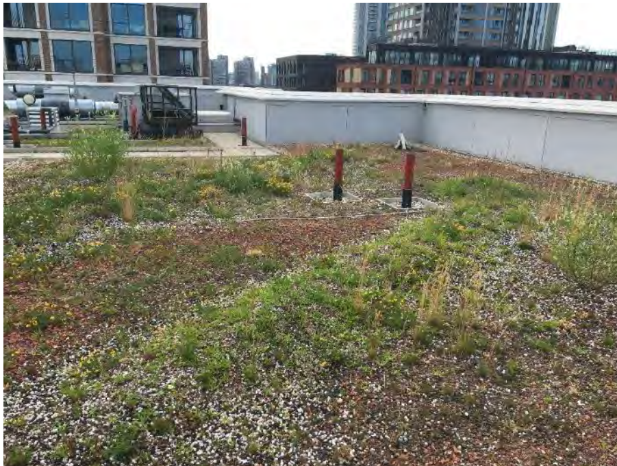
Figure 6.3 Varied substrate depths in situ
