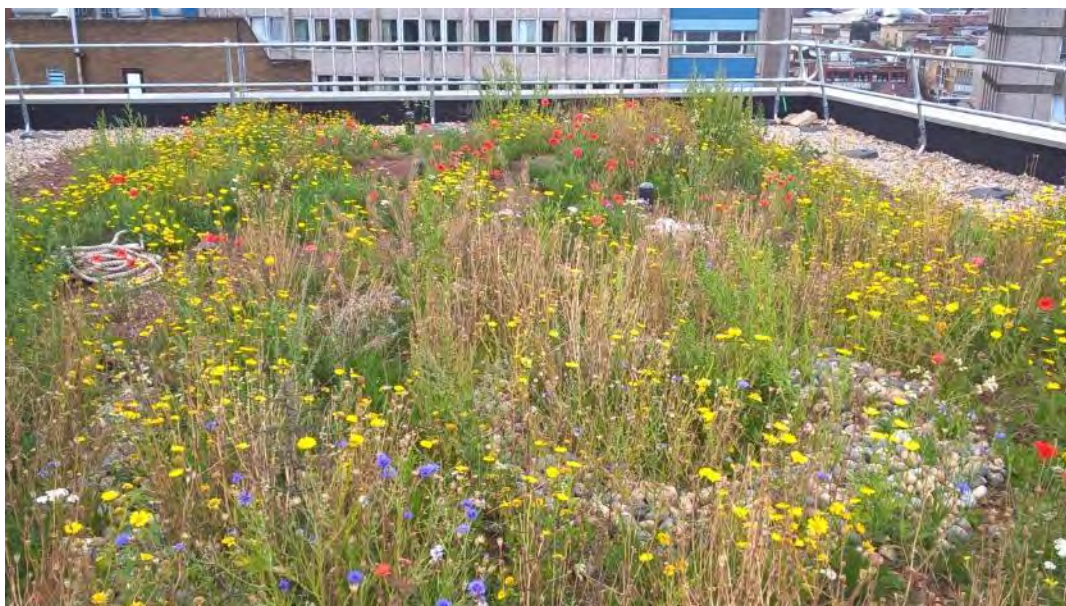
Figure 6.2 Extensive, substrate based biodiverse brown roof in situ.
